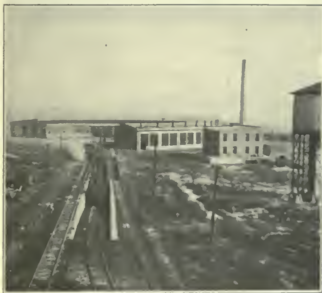
FIG. 346. LOCOMOTIVE TERMINALS. Glenn Yard Locomotive Terminal of the Chicago & Alton Railroad.
